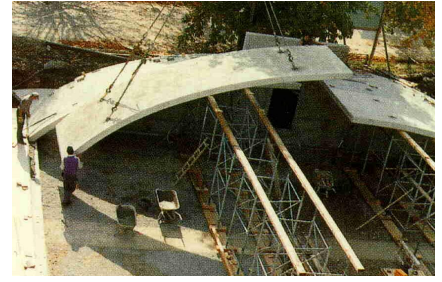
Space saving, flat profile, column free, precast BEBO parking garage under construction in Germany.
