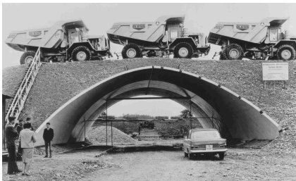
The BEBO 160 mm thick prototype arch demonstrated BEBO's ability to resist extreme loadings.
