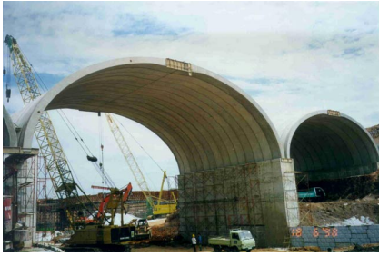
The world's largest precast overfilled concrete arch, an E84T BEBO under construction in Putrajaya, Malaysia.
