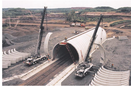
A short, precast BEBO railroad tunnel designed to support high overfills and 500 tonne mining trucks.
