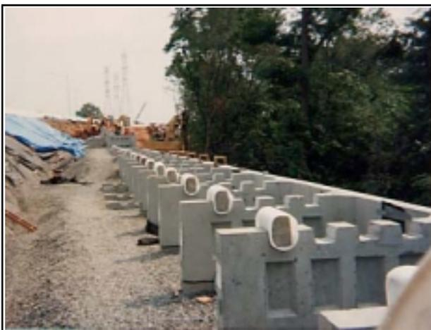
*Shear keys wrapped in joint material*
