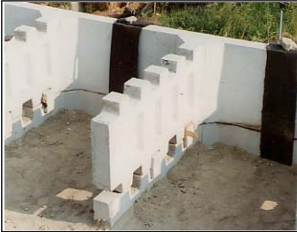
*Filter fabric covering vertical joints on back face*
