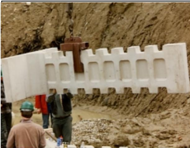
*Lifting a 10' unit at the balance point*
