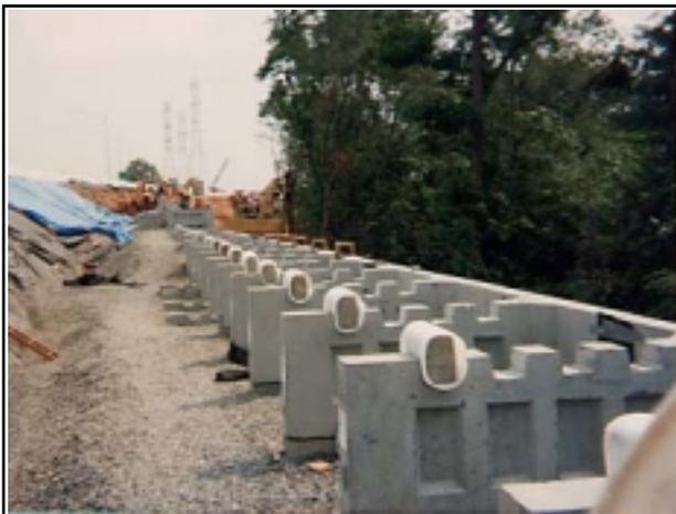
*Shear keys wrapped in joint material*
