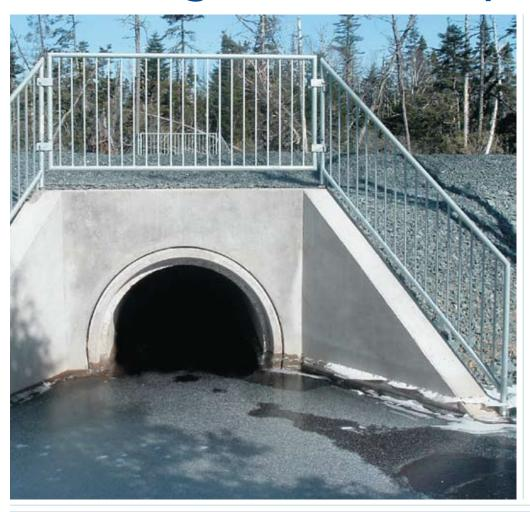
Shaw Pipe is pleased to introduce a full line-up of large diameter precast concrete pipe headwalls to the marketplace this construction season. Shaw Pipe realized there was a market for headwalls that would satisfy stringent municipal and provincial requirements, as cast-in-place concrete is less desirable; construction deadlines are always of crucial importance.
