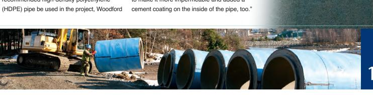
Rylan MacDow, sales manager for Shaw Pipe, says "a very complicated pipe design was required to meet the project requirements, including the manufacturing of the radius pipe, the additional weight requirements to eliminate buoyancy factors, and the special coating and admixtures, all contributed to a very special pipe.
