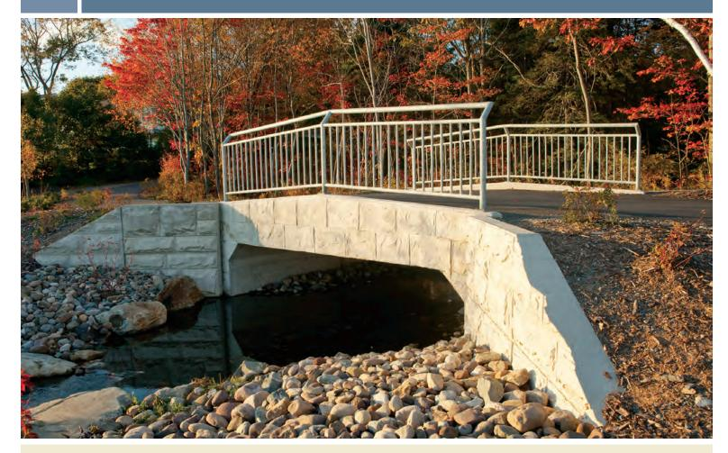
"Shaw Pipe also supplied this four section precast pedestrian bridge and railing, complete with precast curb and architectural veneer finish for the project. The 4300 span x 3600 rise structure serves two purposes. First, it allows pedestrians and maintenance vehicle access to the north side of the lake. Secondly, it permits the 1500mm trunk sewer to cross underneath the natural stream bed."
