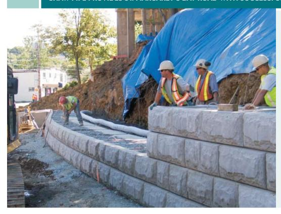
Other characteristics of the wall that required special consideration was the use of Stone Strong Stair Block elements to construct a run of stairs for the entrance to the existing multilevel residential complex. The wall also had to tie in on the opposite end to an existing dry stack stone wall at the same elevation. This was achieved with the use of our 6 square foot radius blocks, which match the existing site contours and elevations.
