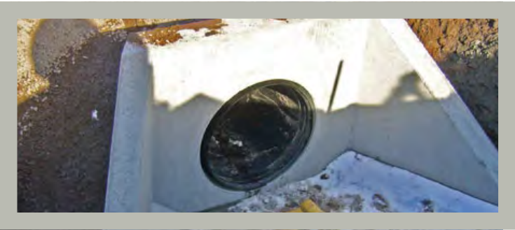
Shaw Precast Solutions supplied 38 special headwall units to the Petitcodiac River Aboiteau rehabilitation. Headwalls required CXL exposure concrete, an increased 300mm wall thickness and A-Lok in-wall gaskets for pipes up to 1600mm OD.
