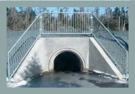
Shaw Precast Solutions 1900x1900 headwall complete with a 1200mm RCP penetration, and Shaw supplied handrail.
