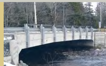
ShawSpan 7.0 meter span with T-Wall wing wall arrangement at Millwood, N.S.
