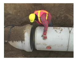
Align the spigot with the bell, ensuring equal clearance around the full periphery, and that the horizontal axes of the two pipes are in-line and parallel. Home the pipe using suitable mechanical means. The homing process will cause the lubricated tube to "roll" over itself, above the compression section, allowing the pipe to "Home"
