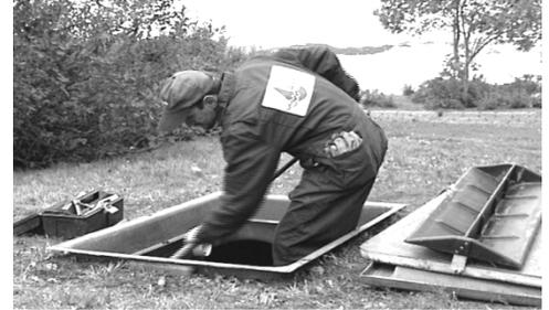
**Annual maintenance performed as per manufacturer's specifications (following manufacturer's requirements)** is essential to ensure the proper operation and performance of your **Ecoflo® Biofilter** and is essential to maintain its warranty on the filter media. Therefore, your **Ecoflo®** must be serviced annually for the entire duration of its useful life. Depending on the local regulation, more than one (1) visit per year may be mandated.
