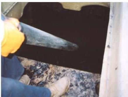
The filter bed is pumped by septic tank pumpers who are authorized by Premier Tech Aqua. The replacement filter must be installed by a Premier Tech Aqua authorized agent.
